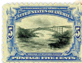
297 Bridge at Niagara Falls
